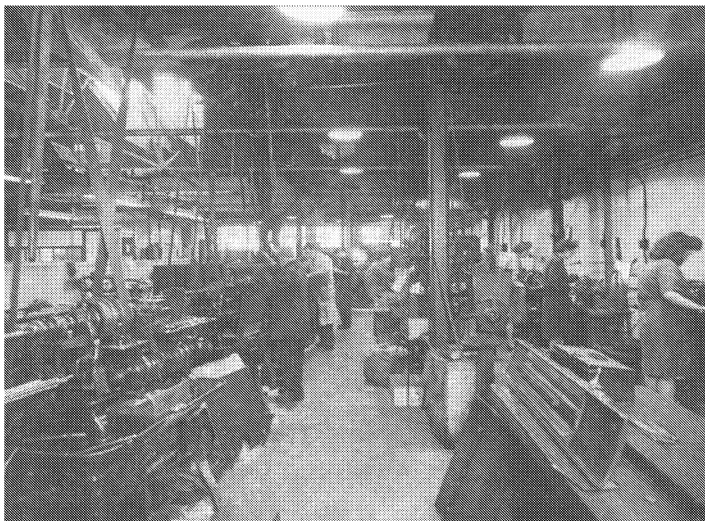
Jacksons' machine shop at Croydon about 1951. Note the belts driving machines from shafting in the roof.
